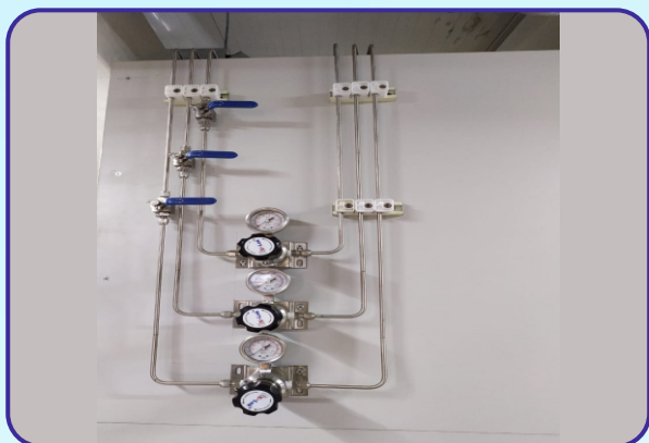
◆ PROJECT GAS PIPELINE WITH LINE REGULATOR
